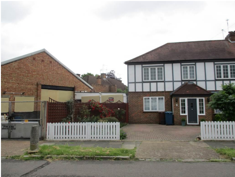
No. 1 Dawlish and application site to the left
